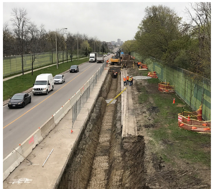
Photo: Replacement of gas lines.
