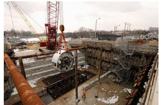
Construction workers lower the first piece of the TBM into the shaft
