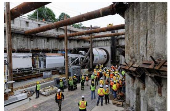
A fully assembled TBM, ready to begin tunnelling
