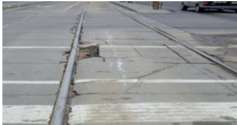
current situation is to replace the streetcar tracks and trackbed. Similarly, the condition of passenger platforms is deteriorating and, at 1.4-1.5 m widths, these are narrower than desirable platform widths. This compromises safety for passengers. The traffic lanes pavement has deteriorated on St. Clair Avenue, with sections due for resurfacing in the next few years.
