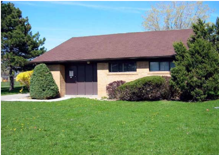
Toronto Hydro Substation in Scarborough
