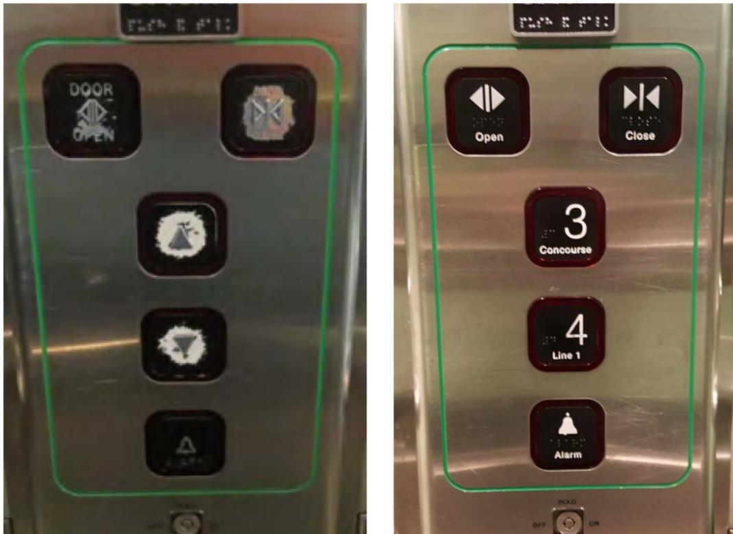
**Figure 3: Original and Modernized Elevator Control Buttons**
